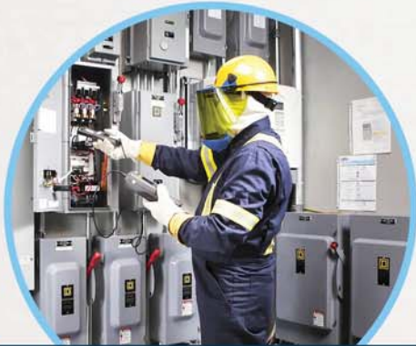
POWER SYSTEM STUDIES
